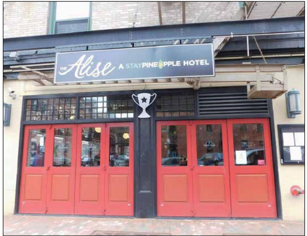
The Alise Hotel remodeled from The Chandler Inn. Photo by Michele Maniscalco
